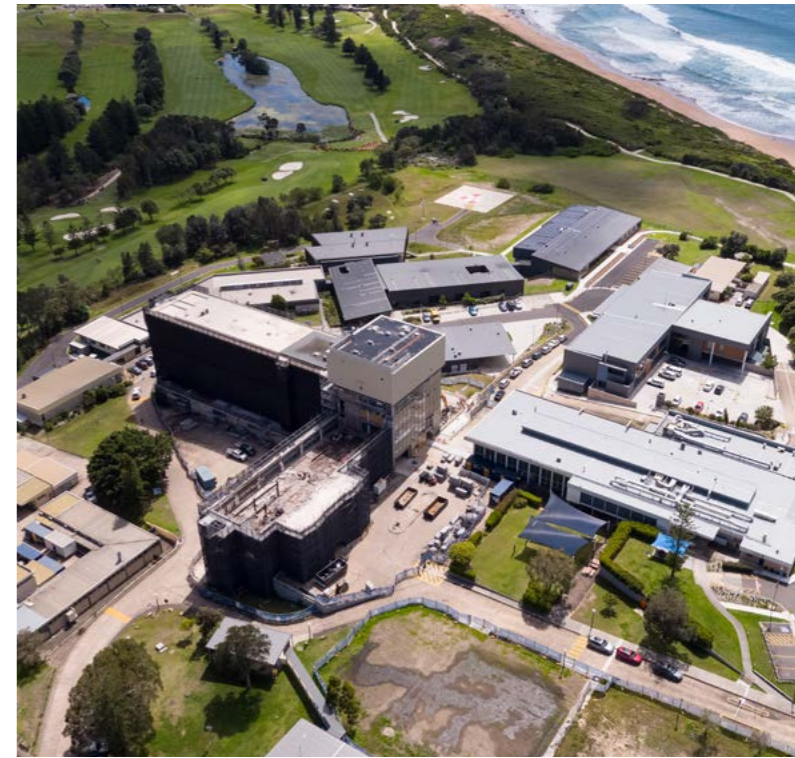
Building infrastructure at Monash Hospital site.
