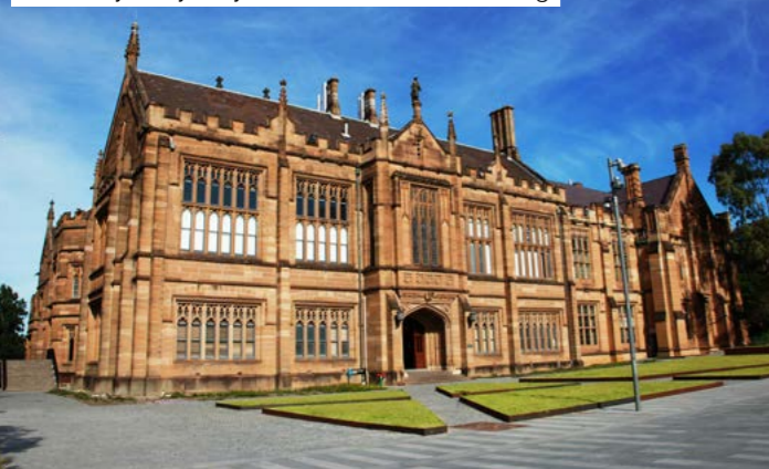
University of Sydney's Anderson Stuart Building
