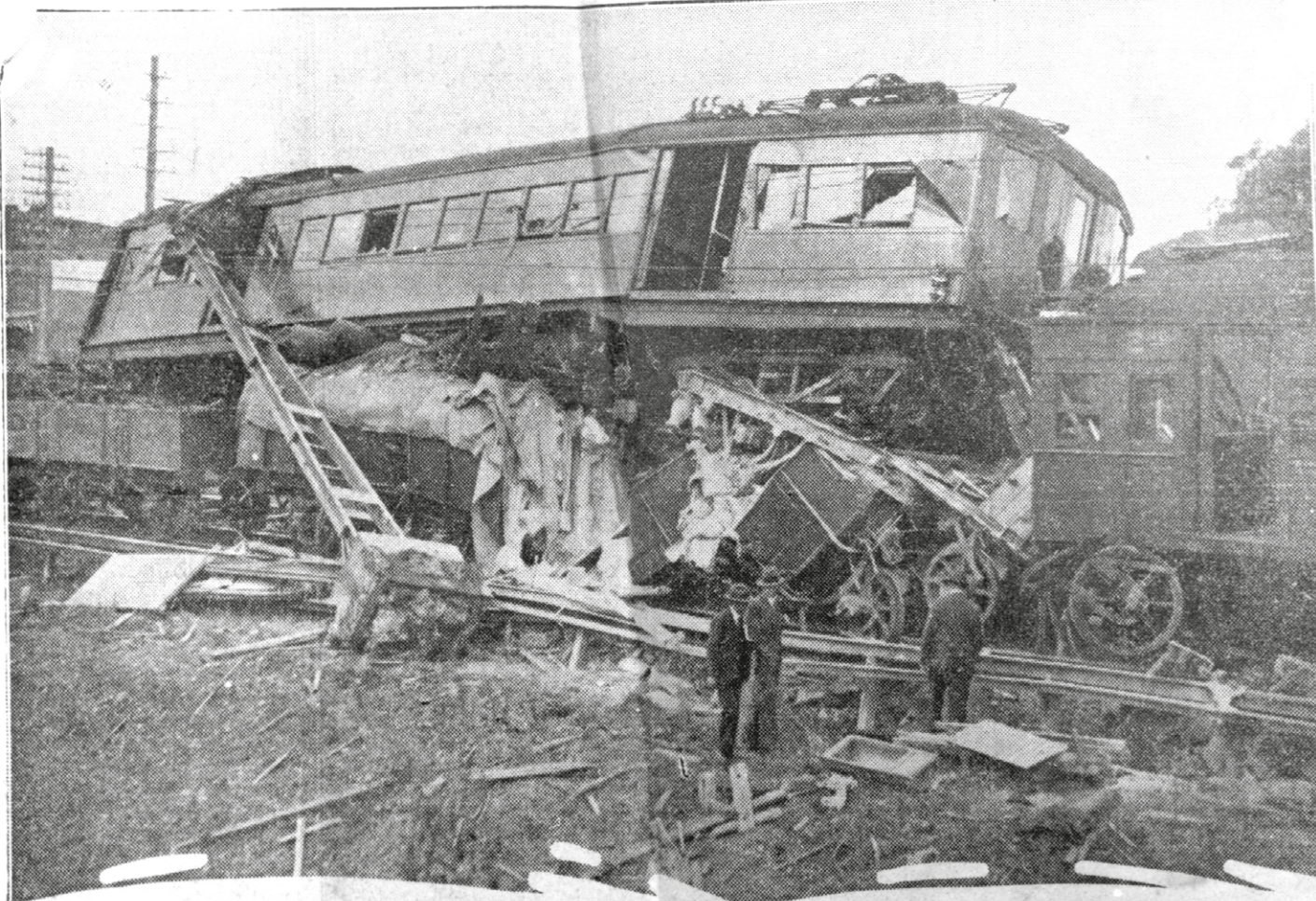
The extraordinary position in which the electric carriage finished after it had crashed into and mounted a stationary goods truck between Pymble and Gordon stations 10-day.
